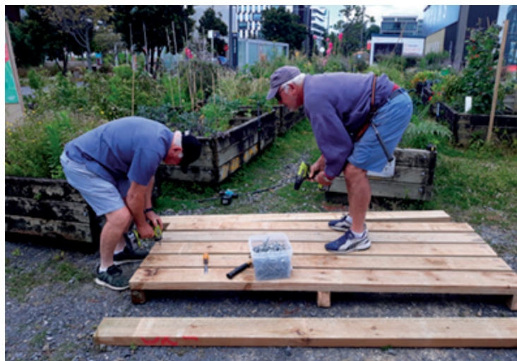
Rex Billington and Alan Foote in construction mode
