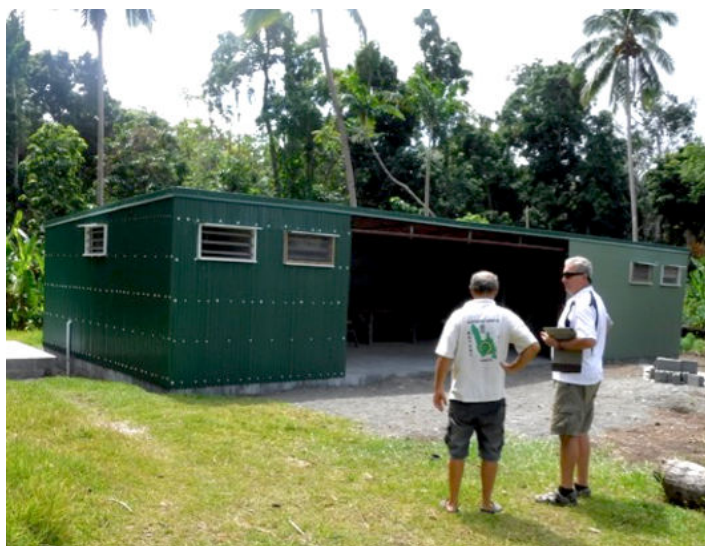
Big Bay water and sanitation project nears completion.
