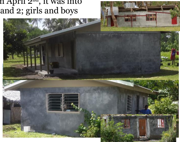
(Photos right above from top to bottom Building 6 (B6) before, B6 after repairs, Building 2 (B2) after repairs and B2 before)
